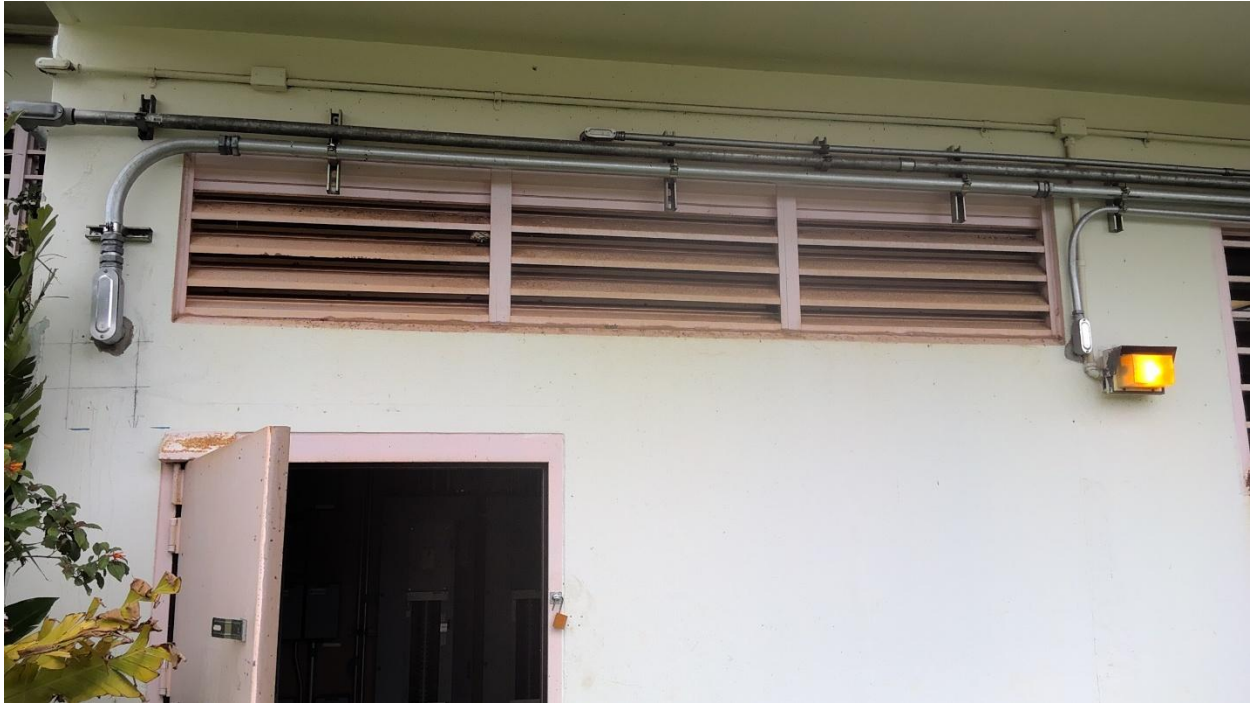
Photo 2 – Top conduit coming into electrical room from outside. Feeds to IT room
