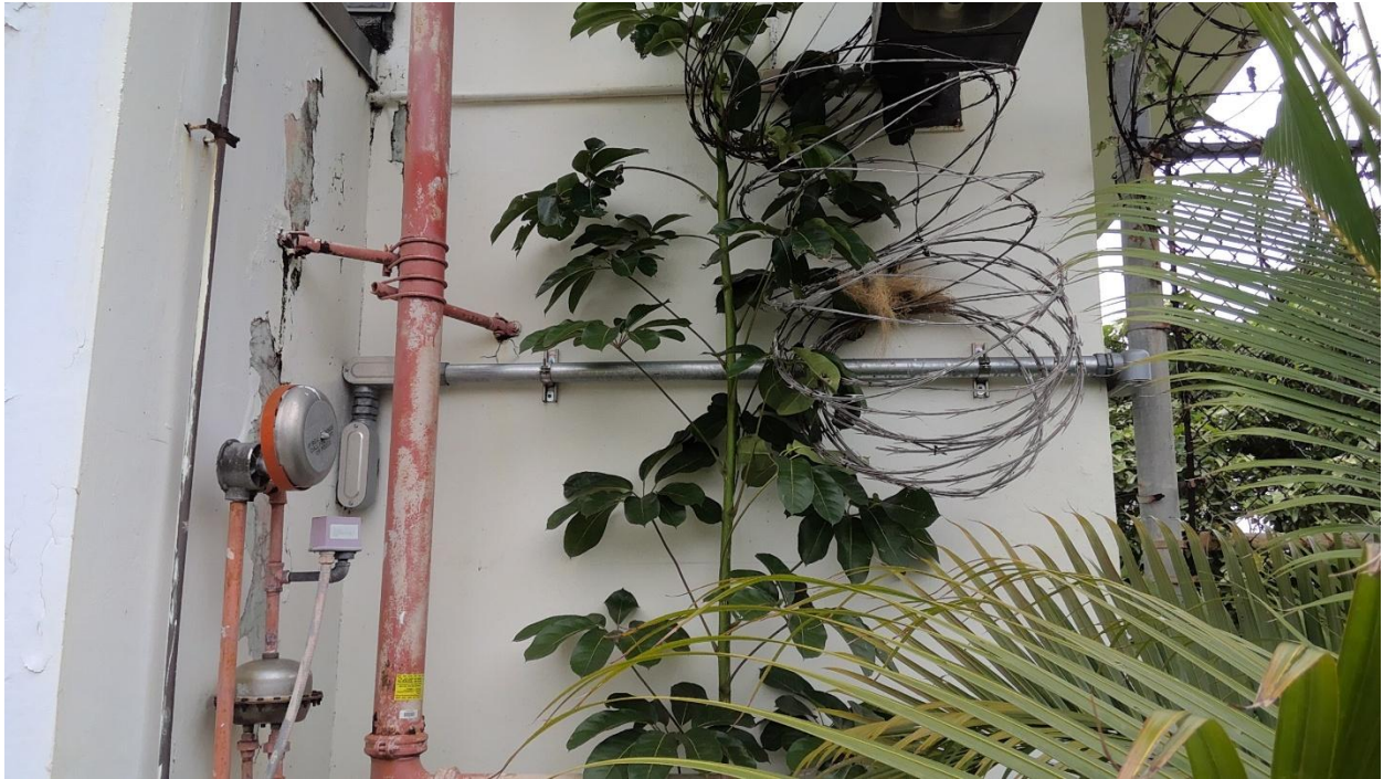
Photo 18 - CCTV Conduit pathway to CCTV poles near Kitchen site
