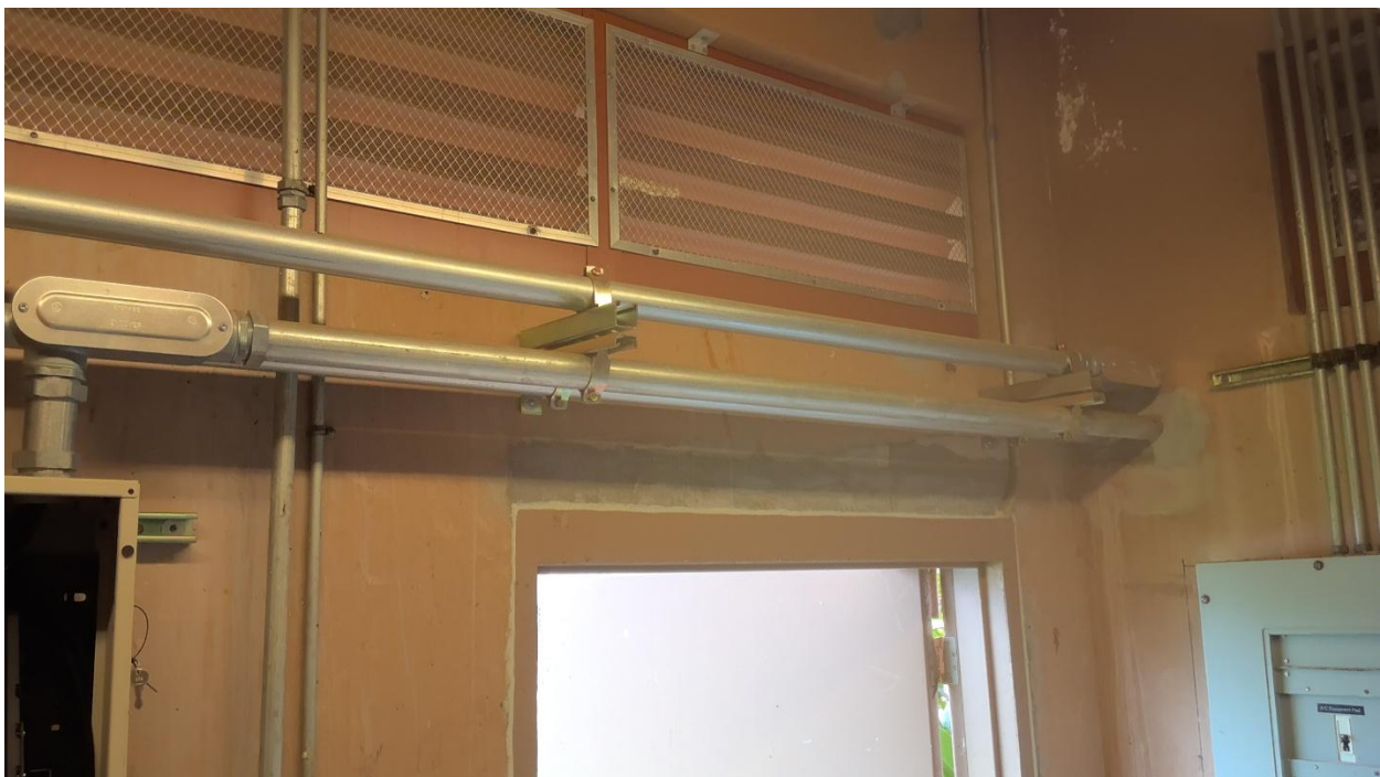
Photo 2 – Top conduit coming into electrical room from outside. Feeds to IT room
