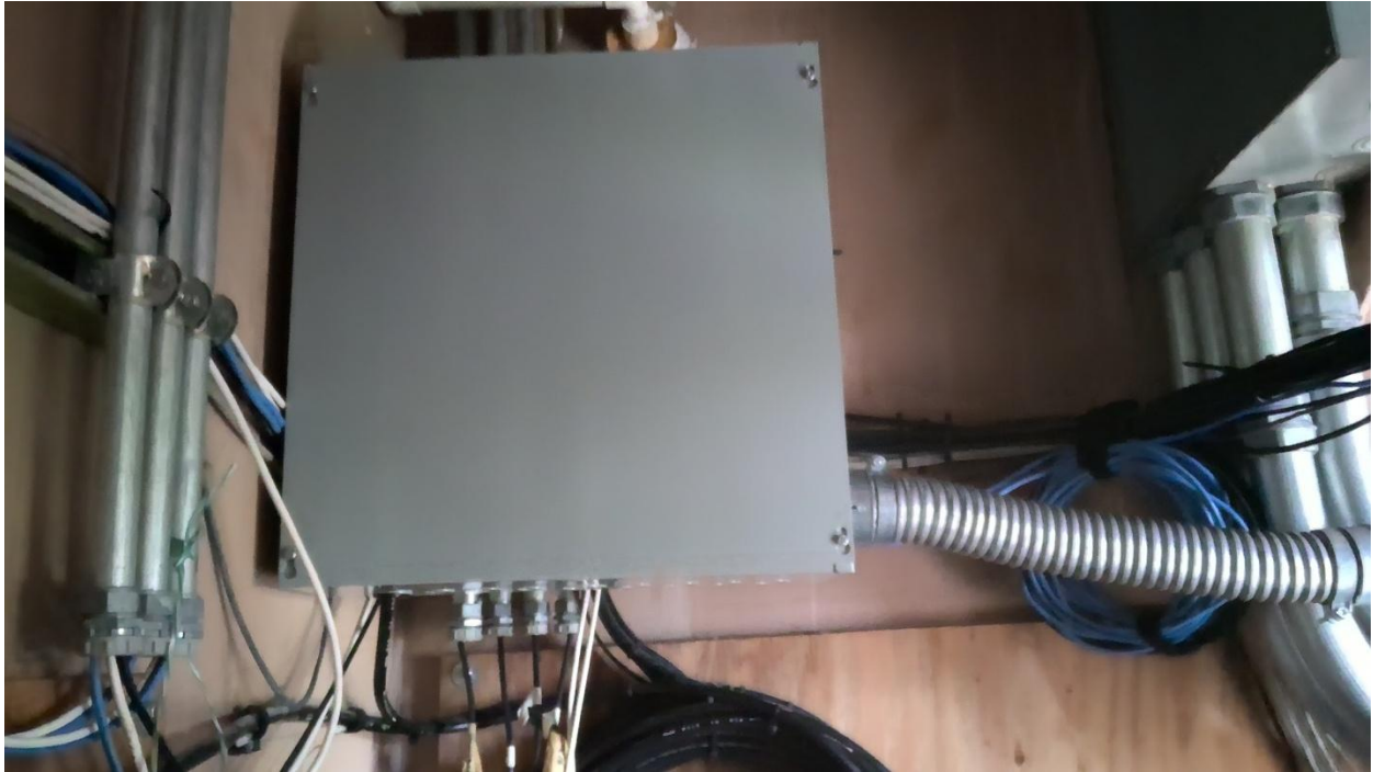
Photo 9 – CCTV panel located in IT room
