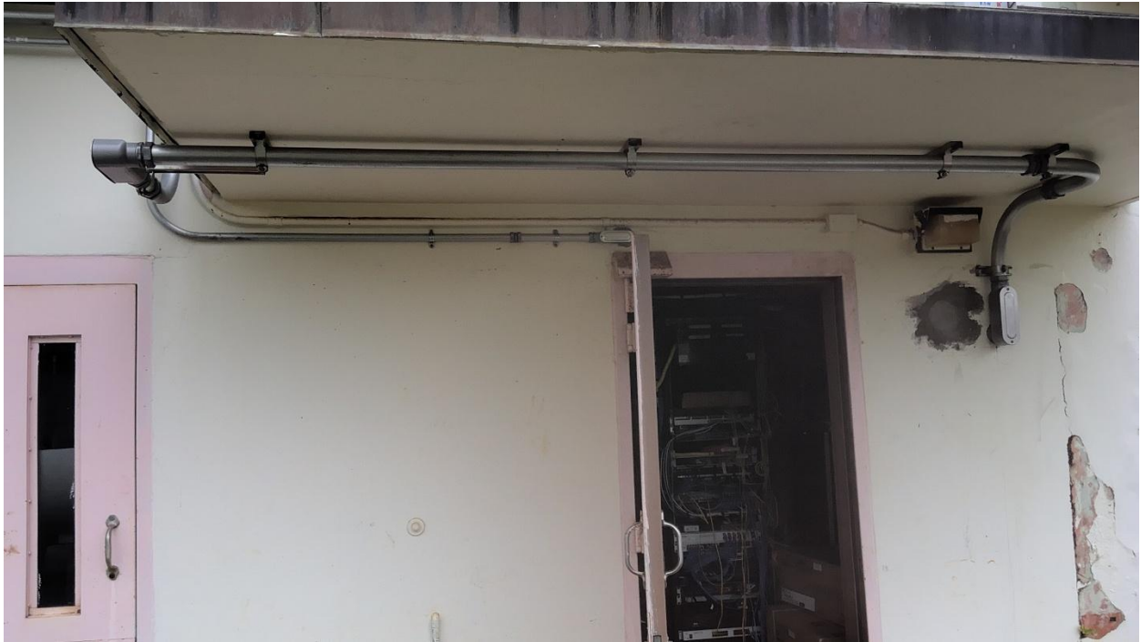
Photo 7 – Conduit from electrical room / CCTV
